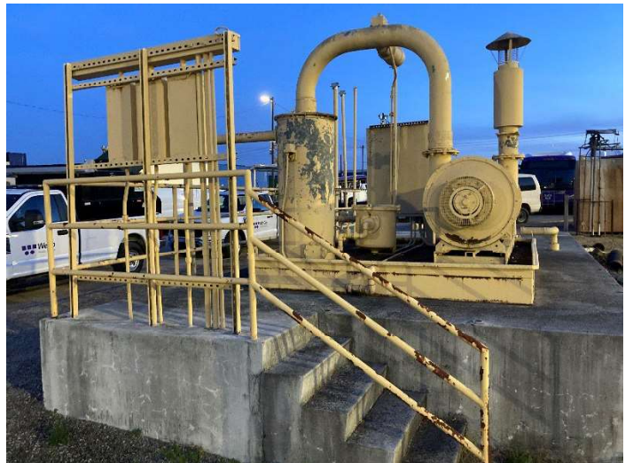
Photo 6: Concrete Pad and Equipment to Be Removed
