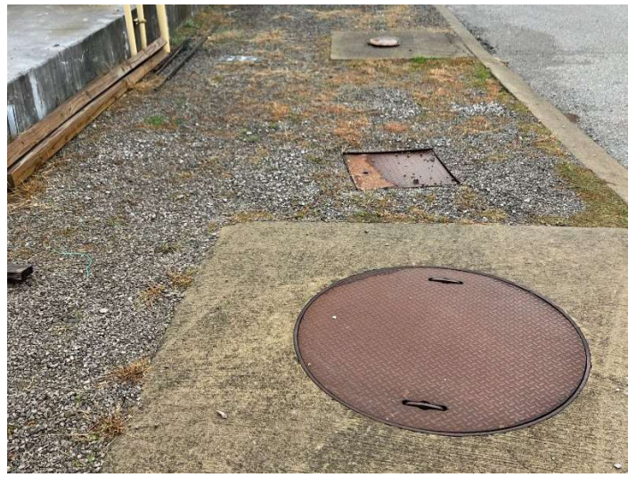
Photo 2: 20,000-Gallon UST (next to concrete slab)
