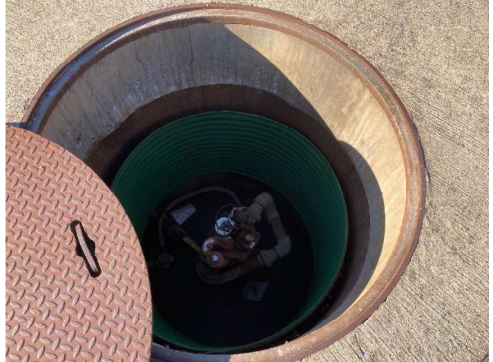
Photo 4: 20,000-Gallon UST Pump Manhole
